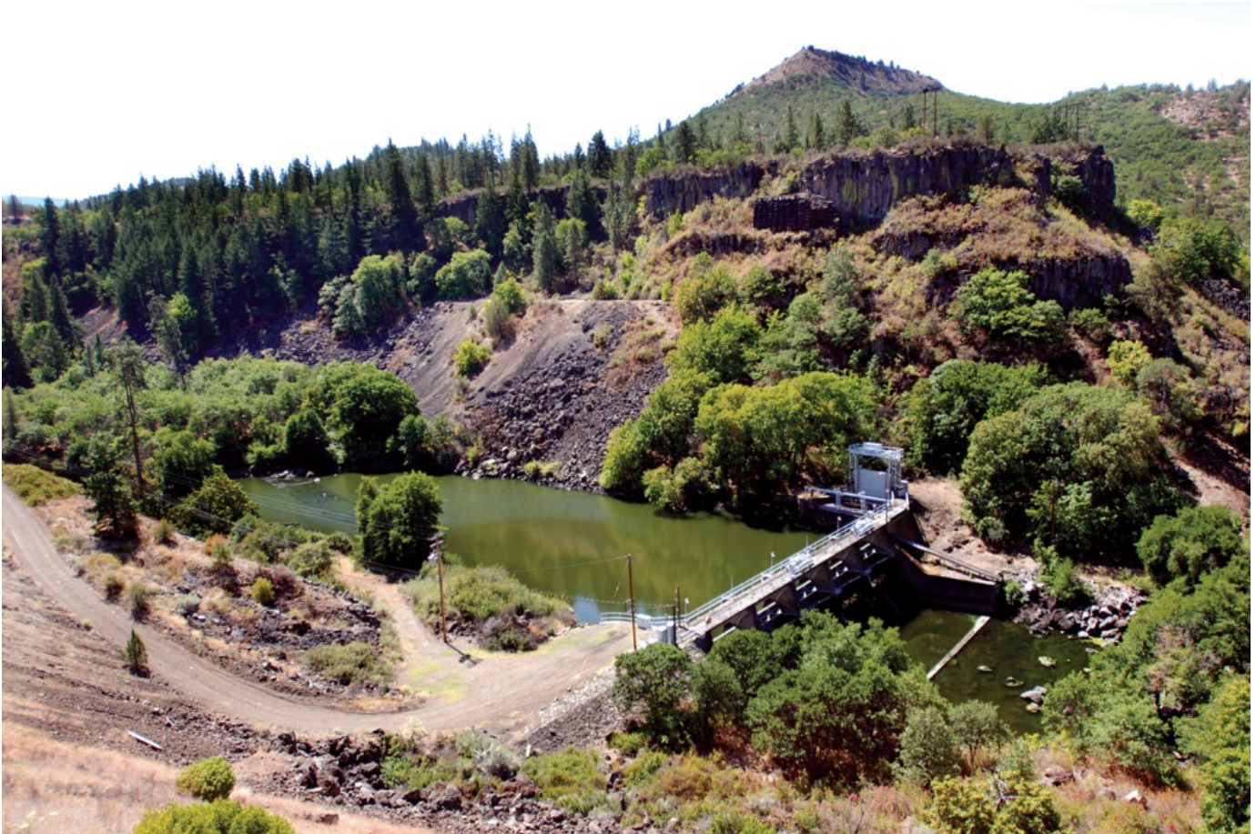
The Copco 2 hydroelectric dam on the Klamath River, outside Hornbrook, California, prior to its removal in July 2023. (AP photo / Jeff Barnard / File)
