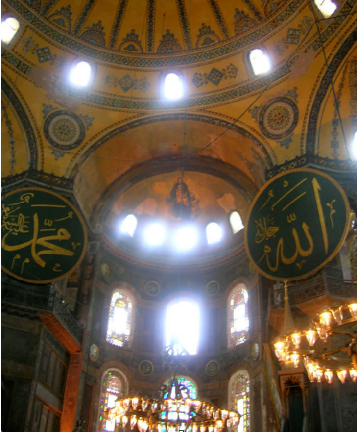
The prime example of this renovation
